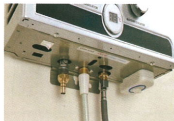
7. Install the water outlet pipe.
