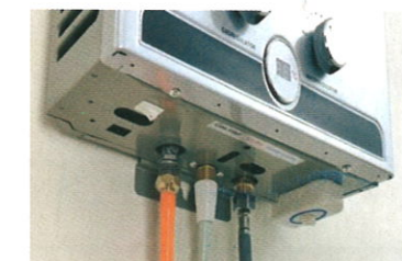
9. Install liquefied gas pipeline.
