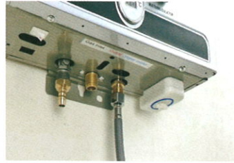
5. Install the inlet pipe.
